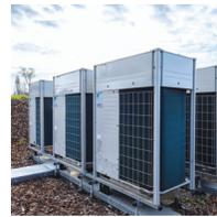
Variable Refrigerant Flow systems take the flexibility and efficiency of heat pump systems to a new level. Not only can they provide heating or cooling without burning carbon fuels, but they can heat and cool simultaneously depending on the needs of different spaces in the building.
